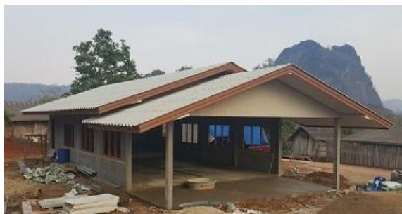
New church building at Jiang Jan under construction
