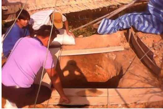
Digging new well
