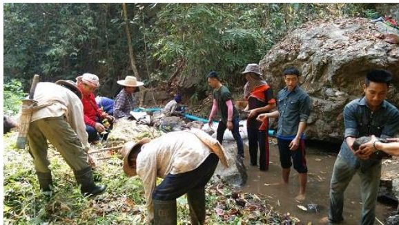
Piping water to the villege
