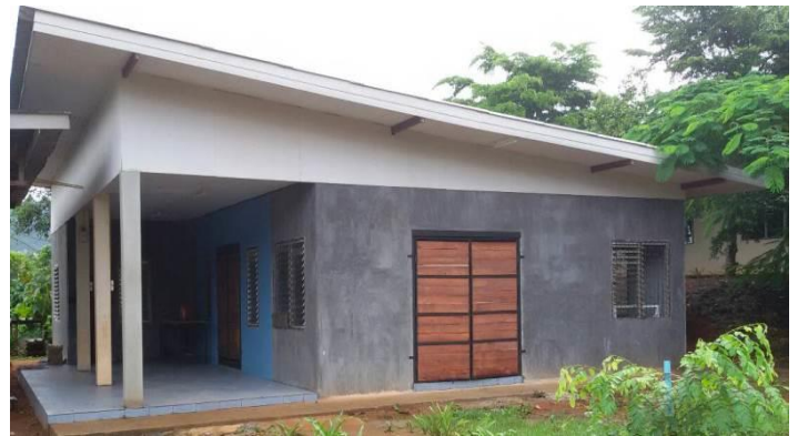
The old church after remodeling
