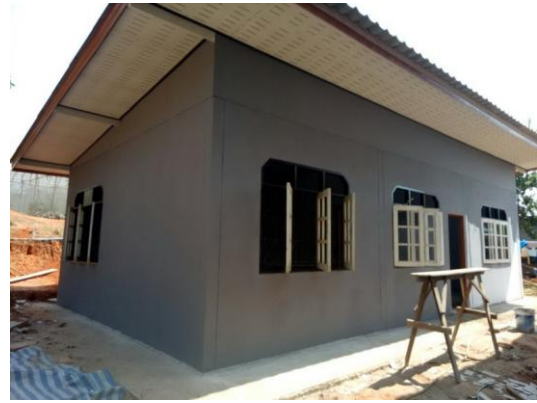
House Parent's new residence under construction
