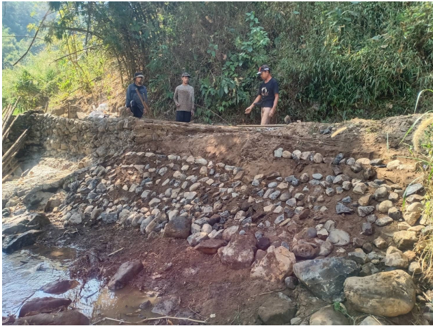
Starting repairs and construction of a stable irrigation canal
