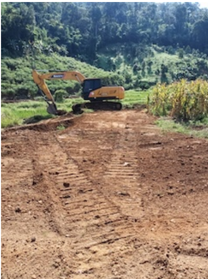
Re-soiling of the damaged rice field
