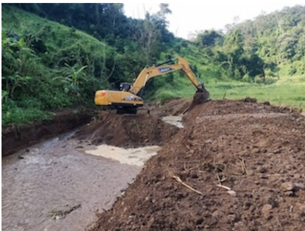
Re-soiling in progress
