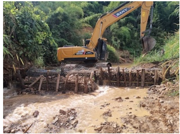
Construction of a new water dam
